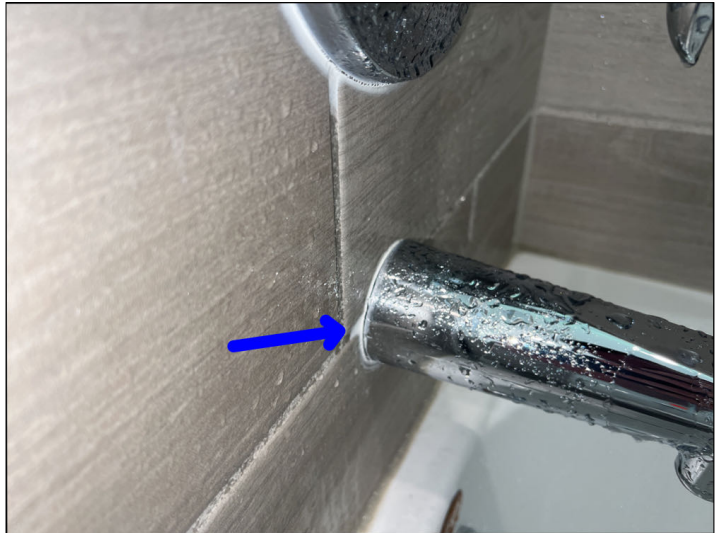
All tub shower faucets and spouts should be sealed to help prevent water penetration behind the fixture.
