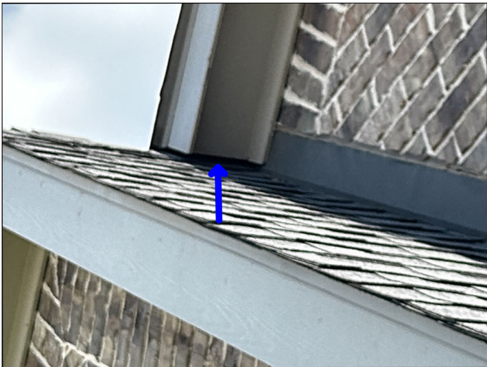
Seal gaps and holes in soffit to help prevent water penetration and rodent intrusion. Mainly at - front
