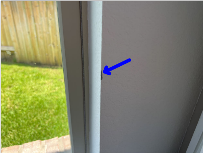
Paint is chipped on the window casing. Mainly at - Right middle bedroom
