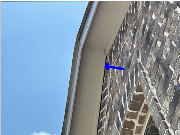
There is loose trim on the home, recommend securing to help prevent future damage and water penetration. Mainly at - front (may be secure but gapped at the ridge of garage)
