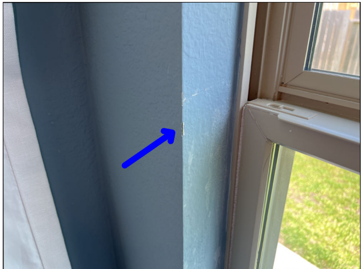
Paint is chipped on the window casing. Mainly at - Formal Dining Room
