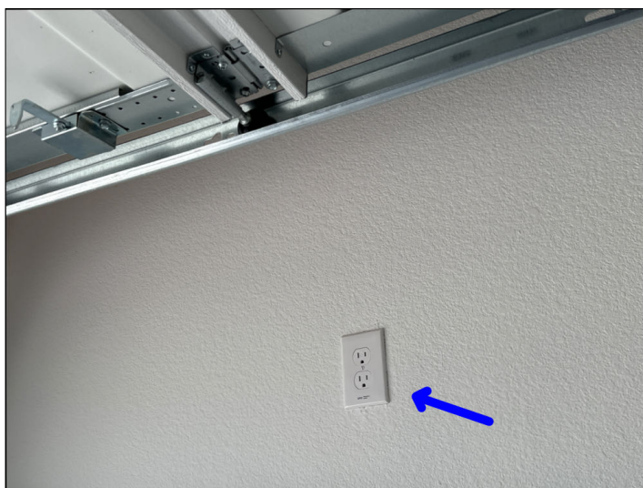
Not GFCI protected above 6' in garage but has a GFCI sticker.
