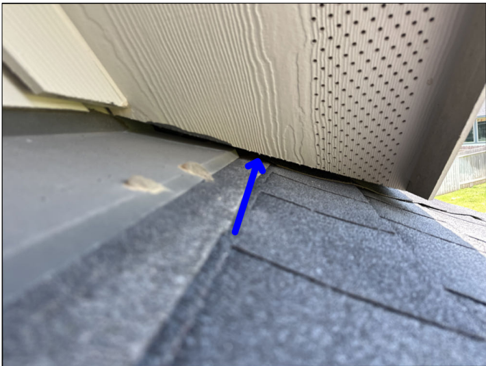
Seal gaps and holes in soffit to help prevent water penetration and rodent intrusion. Mainly at - rear
