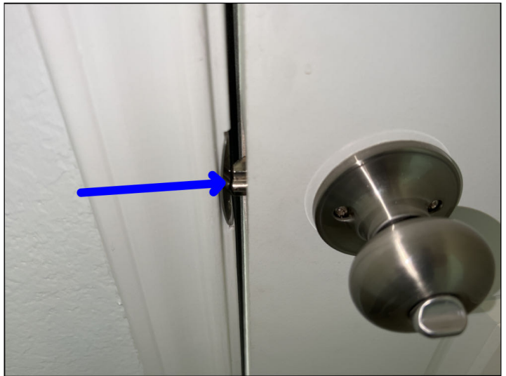
The door latch is not resetting fully, causing the door not to latch in the frame. Mainly at - Garage entry
