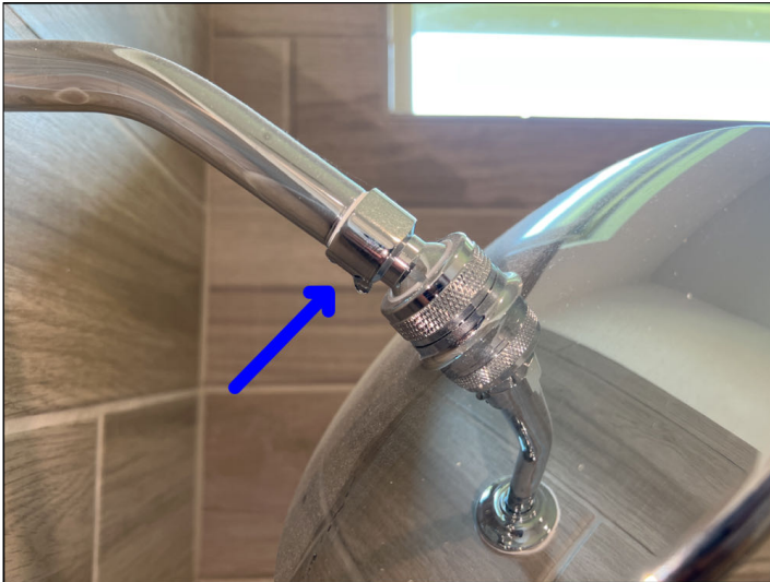
The shower head leaks at the connection. Mainly at - Hall bath
