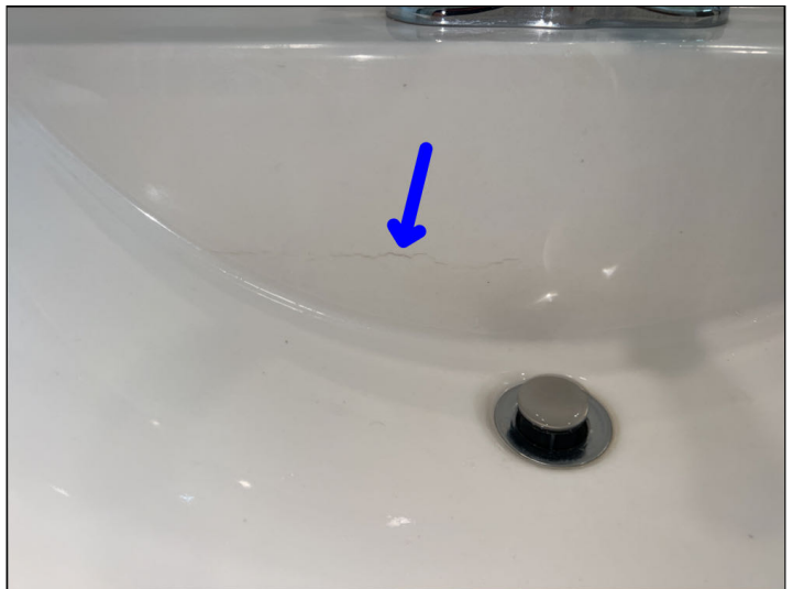
There is a crack noted in the sink which could potentially lead to a leak beneath the sink into the cabinet. Mainly at - Hall bath
