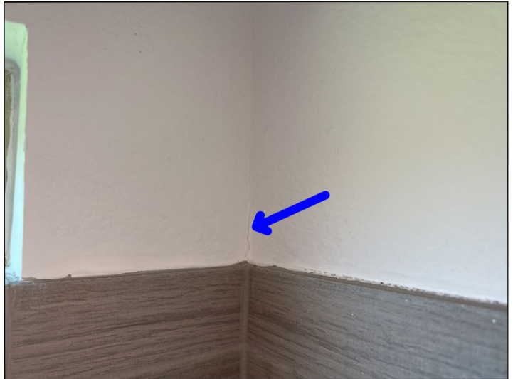
Settlement cracks were noted in the drywall. Mainly at - Hall bath
