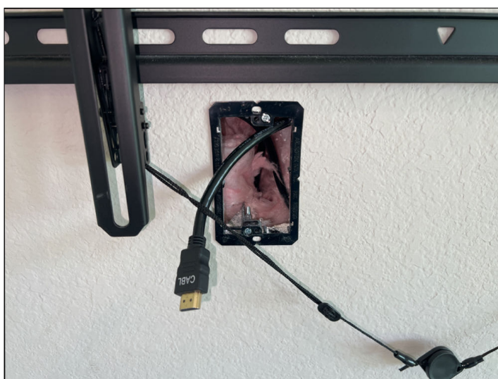
Low voltage cover plate is missing. Mainly at - Living Room
