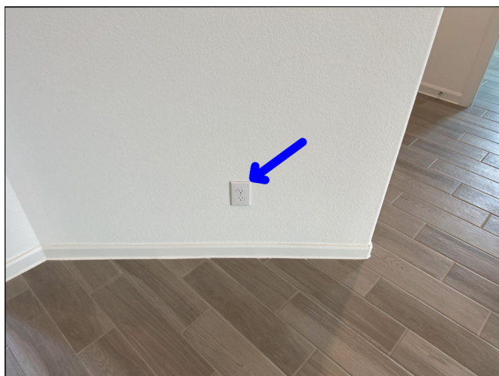
The receptacle is loose. Mainly at - Front Entry
