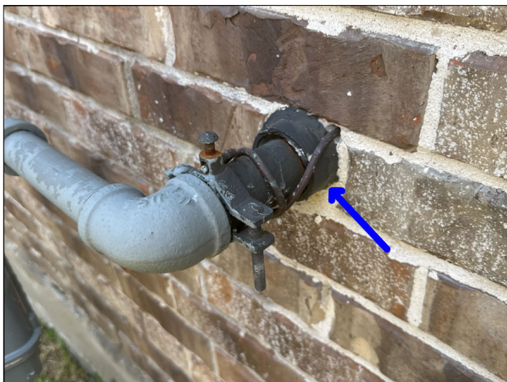
Bonding was noted on the gas line as recommended.
