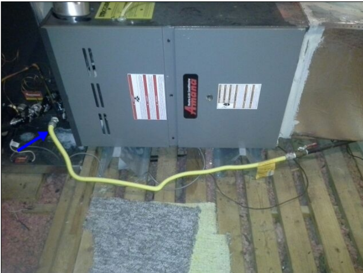
There is no drip leg or sediment trap for gas line on the furnace. This helps prevent trash from clogging jets.
