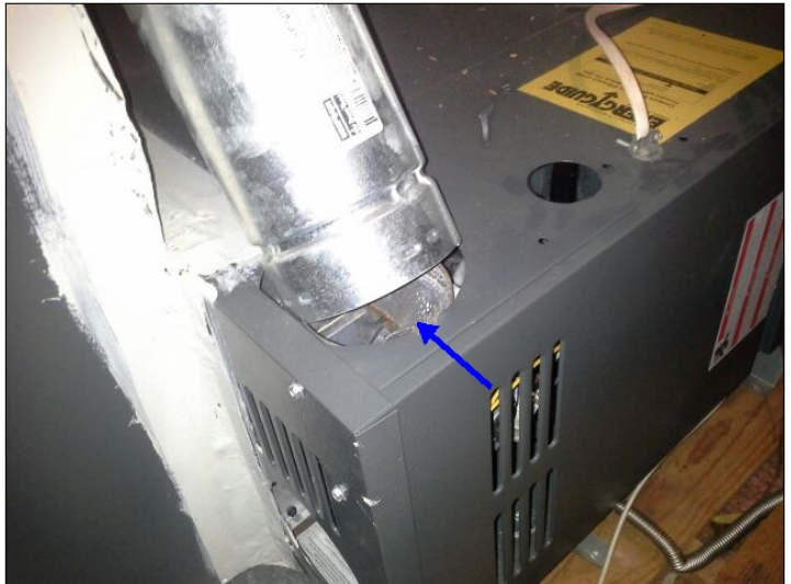
The vent pipe for the furnace is loose or separated causing a carbon monoxide to leak in the surrounding area. This can be dangerous or fatal if not corrected, recommend a heating specialist for immediate repairs.
